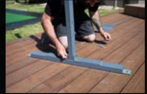
STEP 4: using 2 x bolts & washers, bolt each floor plate to the upright
