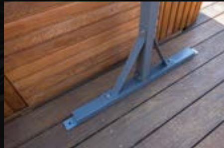
STEP 10: stand awning up & ensure square before fastening to ground/deck or dyna bolt (not supplied) into concrete
